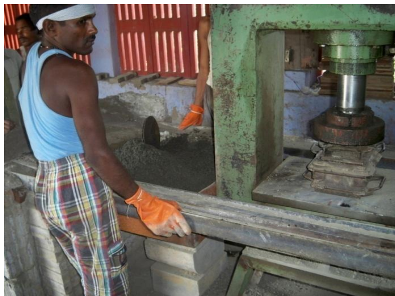
Figure 4.5: Casting of Tiles
