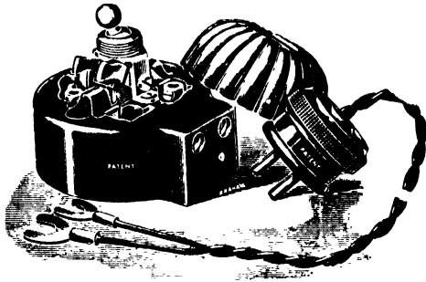
FIG. 77.—A Charging Switch for dealing with small car batteries.
