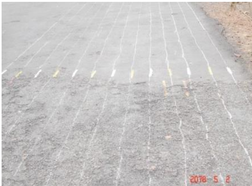
Plate 4.4: Marking Over Entire Width of the Pavement
