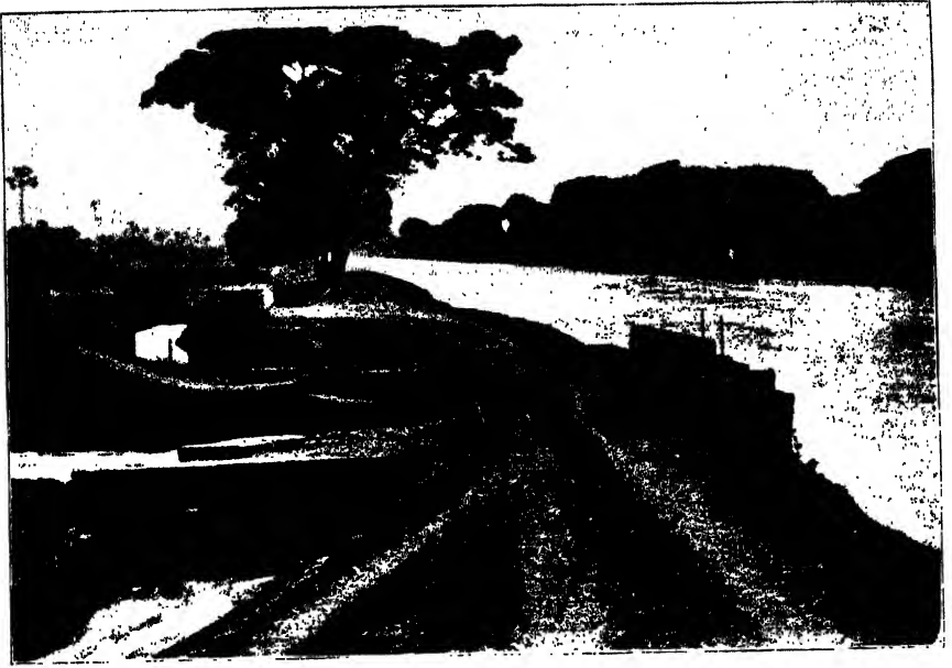
CANAL IRRIGATION IN GODAVARI DISTRICT.
