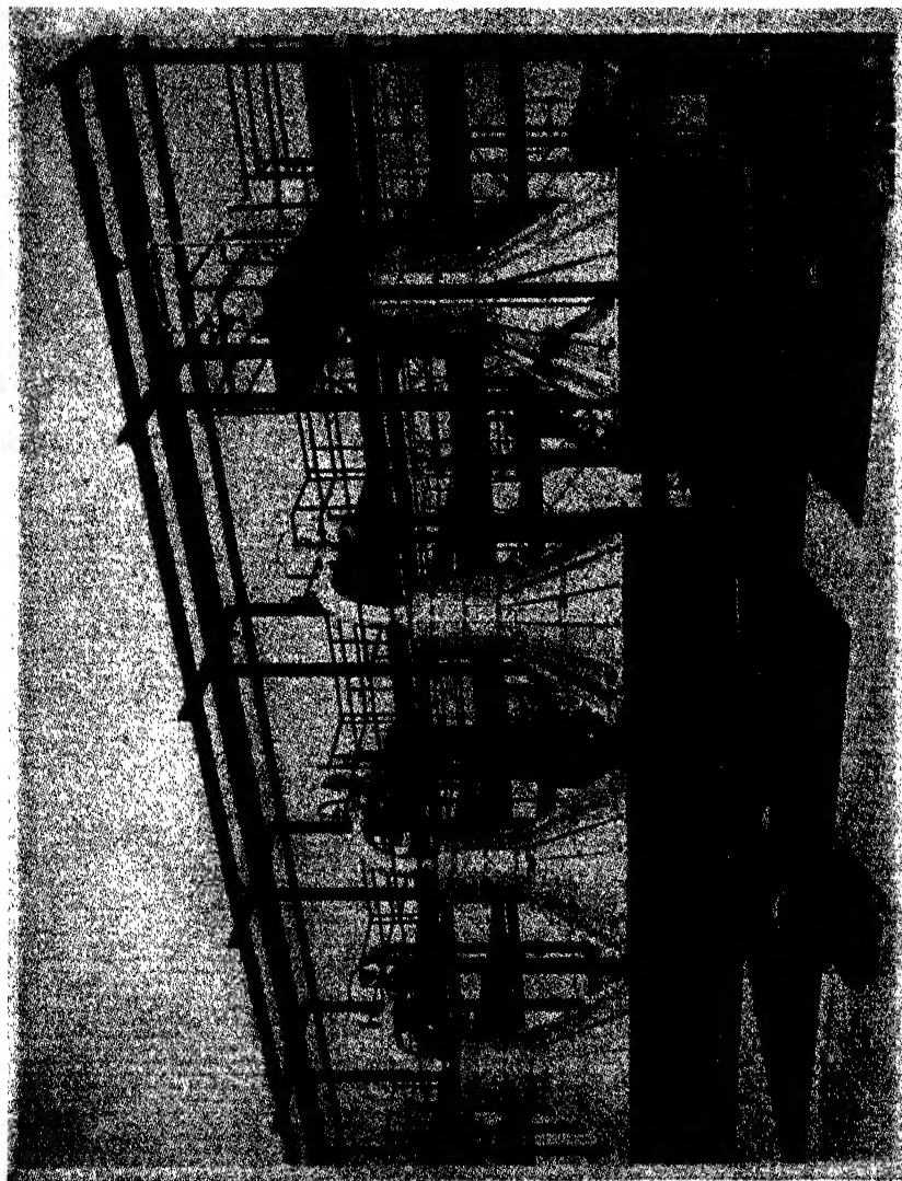
FIGURE 6. A Plant of Four Simonson-Mantius Vacuum Sulfuric Acid Concentrators. Capacity, 80 Tons of 65° or 280 Tons of 60° Acid per day.
