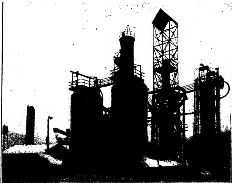
FIGURE 18. Two Gray Process Towers in Series Directly Connected with Dubbs Cracking Unit.
