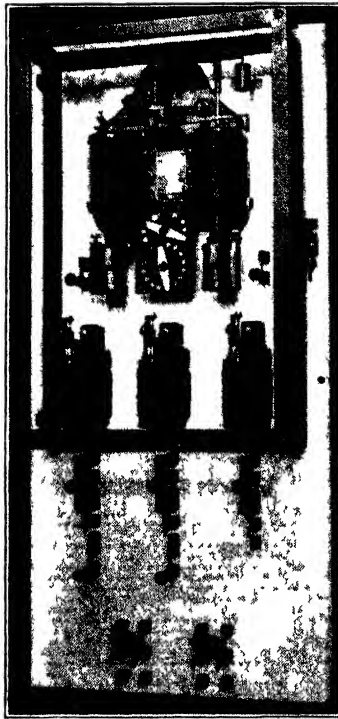
Fig. 47 Westinghouse Type A Voltage Regulator Panel
