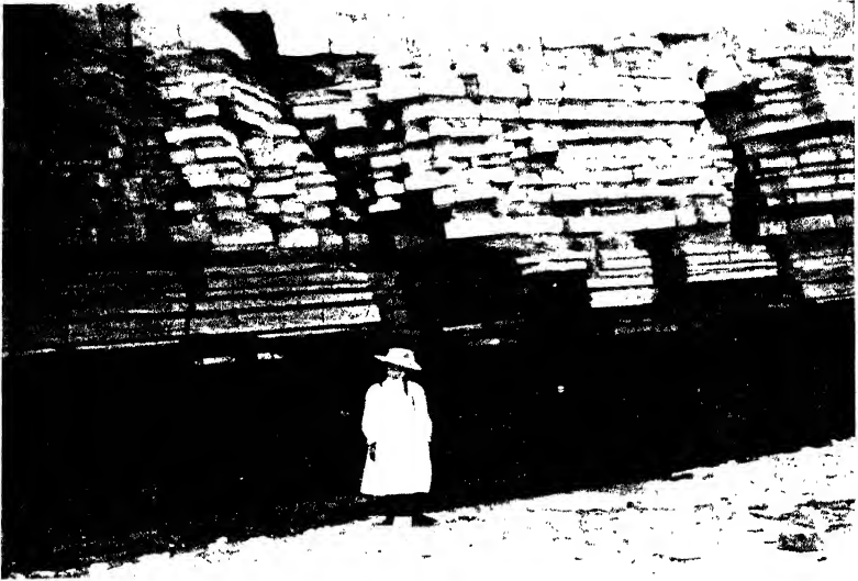
(a) Bedding and joints Limestone and shale of the Lower Lias, Penarth
