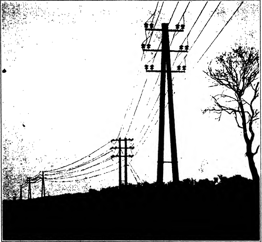
FIG. 40.—Good example of ordinary road-crossing and angle in the line. Two circuits each 3—0.1 sq. in. bare copper strands and a continuous earthed guard wire located below. 35,000 volts. With proper size, use, and construction of one continuous earthed guard wire, a double three-phase 3-wire line as shown here could be converted into two three-phase 4-wire circuits delivering many times more power, be safer, more reliable, cost practically the same, and have an earning capacity very much greater.
