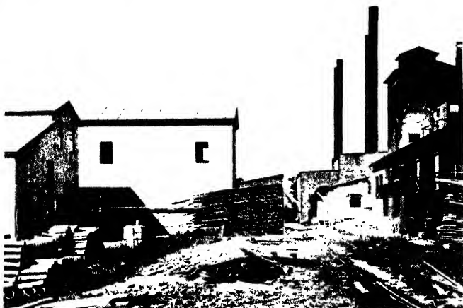
Dow Chemical plant, Aug. 31, 1900. Above shows rear of decomposer houses and in rear site of original bromine plant: below, to the left, is the lime house; and to the right, the power house and the warehouse.
