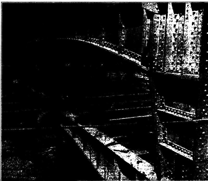
FIG. 47. Erection view of ramp-type garage, Cincinnati, Ohio, showing beam and girder construction. (Courtesy of American Bridge Company.)
