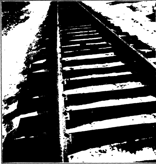
FIGURE 36. Hewed cross ties laid 26" apart, center to center, on the tracks of the Boston and Maine Railroad in Maine. Note the tie plates used to increase the bearing surface and to prevent the rail cutting into the wood and the use of single-nail spikes. Some railroads formerly used the screw spike. The prevailing practice is to use tie plates with nail spikes.
