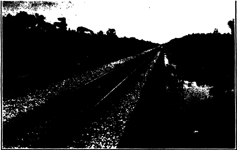
FIGURE 42. Section of the 2-mile double-track ballast-deck creosoted-timber bridge built by the Illinois Central system over the Bonnet Carre spillway near New Orleans in 1935. More than 10,000 creosoted piles, totaling 850,000 lin. ft., and 4\frac{1}{2} million b.f. of creosoted timber were required for construction of this bridge. The cross ties are also creosoted.
