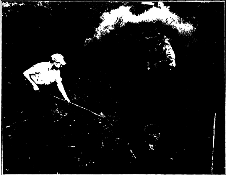
FIGURE 135. Drawing a charcoal pit in southern Ohio. The charcoal is being raked away from the slowly burning pile. This charcoal pit has burned for 7 days and is about one-third its original size. In this section the average pit is made with 25 to 30 cords of hardwood and produces about 1000 bushels of charcoal. Each cord of wood produces about 33\frac{1}{3} bushels of charcoal. Each bushel weighs 20 lb. Courtesy U. S. Forest Service.
