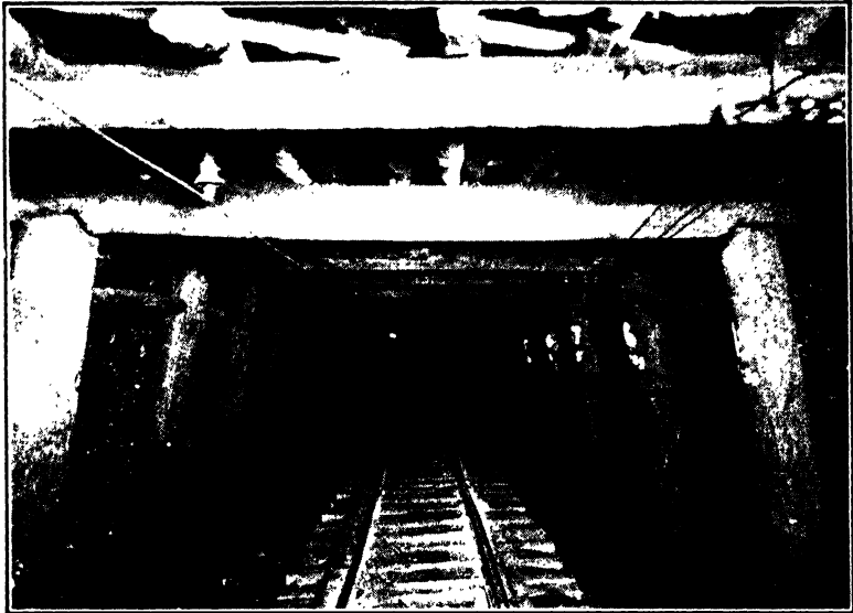
FIGURE 62. Typical view in anthracite mine in Pennsylvania, showing props, caps and lagging, and mines ties.
