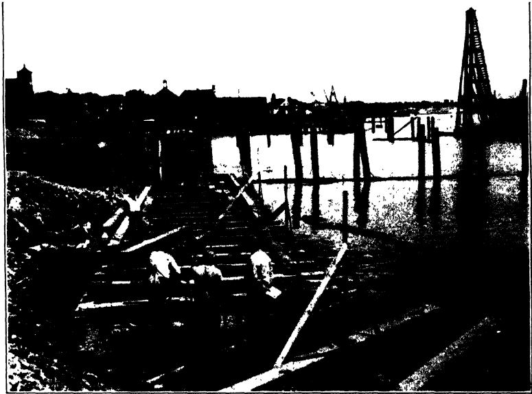
FIGURE 44. Piling used in harbor improvements along the Potomac River at Alexandria, Va. At lower left is shown a relieving platform supported by piling. Various types of ferry slips, piers, wharves, and abutments are constructed of or supported by piling. The familiar pile driver is shown at upper right. Courtesy U. S. Forest Service.
