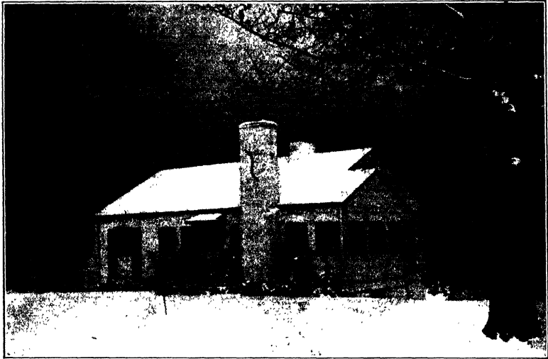
FIGURE 30. Typical Gunnison home, prefinished with plywood outside and inside, plywood floors and partitions as well as plywood base for roof. Made in complete prefinished units at the factory, ready to bolt together on foundation at the site. Modest decorative exterior features added to conventional design as shown. Courtesy Gunnison Homes.
