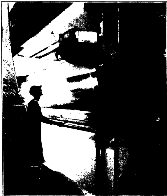
FIGURE 74. Paper passing through dryers at high speeds to remove the last vestige of moisture. Rolls are steam-heated. Courtesy Mead Corp.
