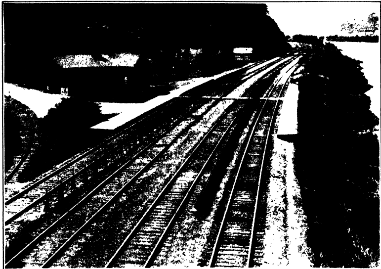
FIGURE 34. Main line of Pennsylvania Railroad with its 4-line right of way and well-ballasted track with treated ties at Stoopes Ferry, Pa. The Nation's railroads which pioneered in the use of pressure-treated ties are now turning to the economy of treated wood for cars, grade crossings, poles, and general construction.
