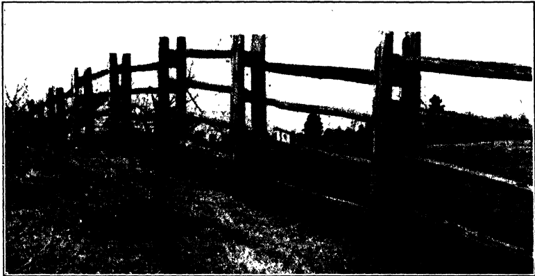
FIGURE 51. One of many types of wood rail fences as used near Rapid River, Mich. Fence posts are one of the most important uses of forest products. The old rail fences have almost disappeared in favor of wire fences, particularly in the western range country and along railway right of ways. The posts and many of the rails are of northern white cedar. Rustic forms of rail fences as shown here have recently come back into wide favor. Courtesy U. S. Forest Service.
