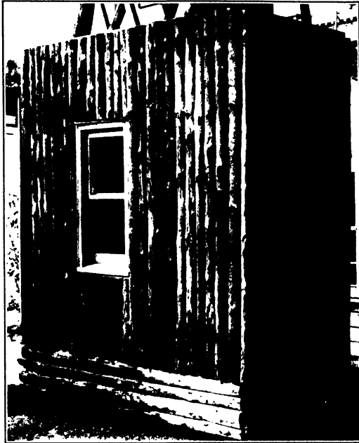
FIGURE 153. Exterior corner of log cabin. Siding made from thinnings from a 32-year-old Norway spruce plantation in New York. Top diameters of 9' logs were from 5½" to 6½". The 25 logs were equivalent to 50 cu. ft. or about ½ cord. As sawed these logs produced 282 b.f. of 2" log-cabin siding and 78 b.f. of lumber. Courtesy H. L. Henderson.
