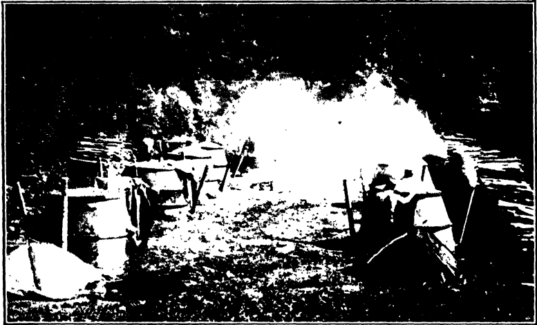
FIGURE 136. The Black Rock Forest portable charcoal kiln, as developed by Tryon in New York. This shows 12 kilns in operation, wood ranks on left and right, brick floors, and kilns cooling while others are being loaded and in process of burning. Photograph by H. H. Tryon.
