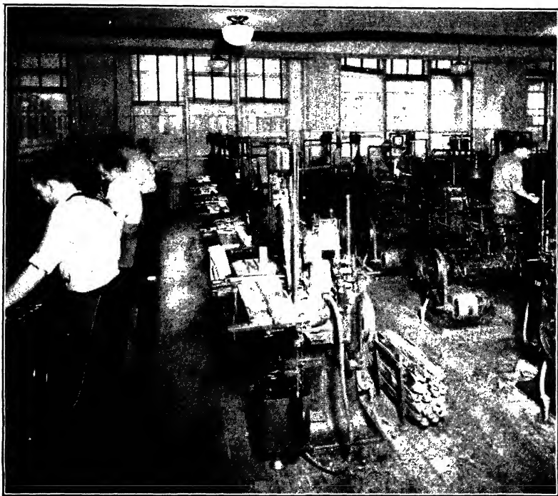
FIGURE 5. General Ventilation in a Printing Plant
