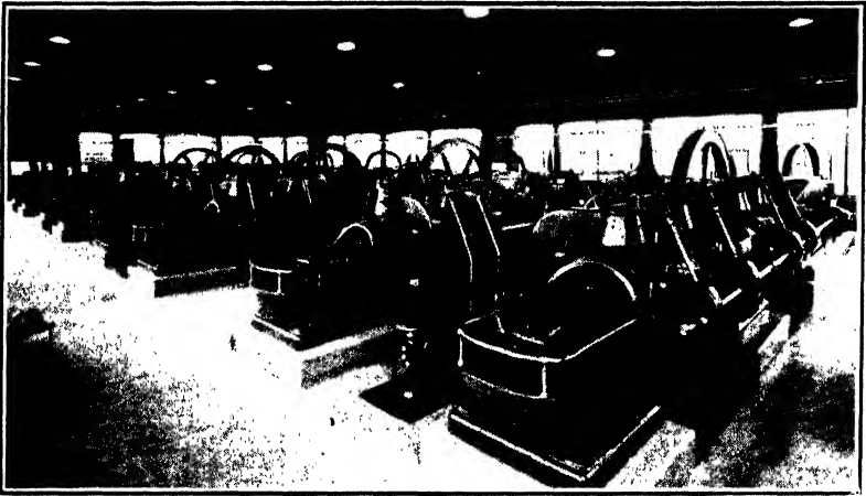
FIG. 35. Gas compressor station with 5 four-stroke cycle twin-tandem double-acting gas engines driving single-stage compressors for boosting natural gas pressure from 165 to 450 lb. Engines use water-cooled floating pistons.
