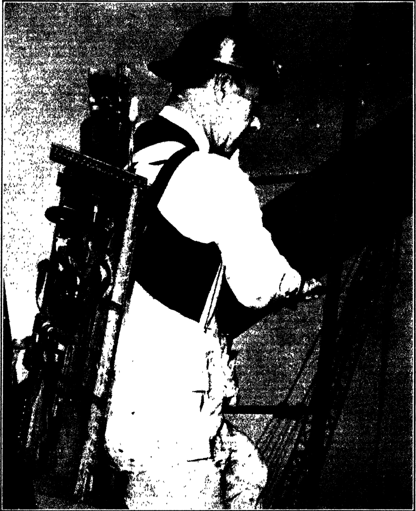
FIG. 83. Special tool rack used at the Kaiser Company shipyards contains all tools needed by the joiner, yet his hands are free enabling him to climb up and down holds.
