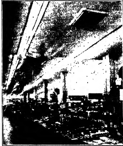
FIG. 258. Concentric-ring air diffuser.
