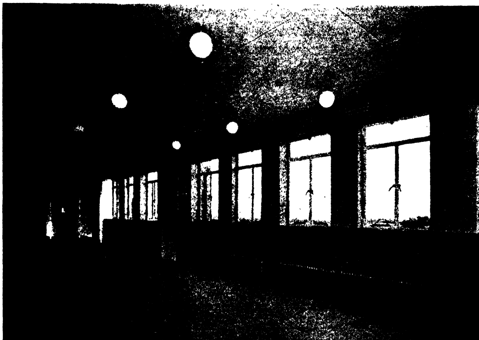
FIG. 43. CANTEEN IN A LONDON FACTORY SHOWING DIRECT HEATING AND INLETS FOR TEMPERED AIR SUPPLY AT HIGH LEVEL
