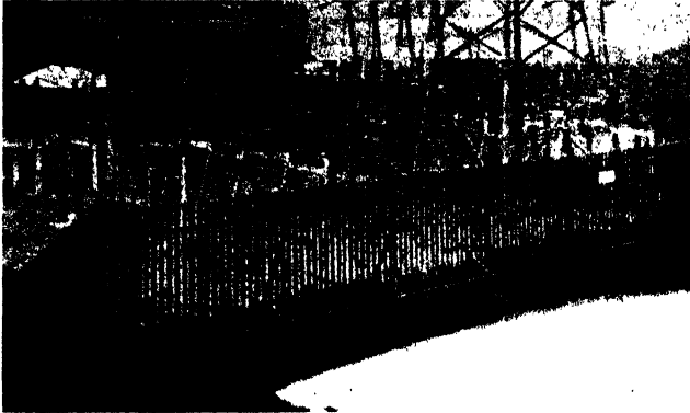
FIG. 17. UNCLIMBABLE STEEL FENCING
