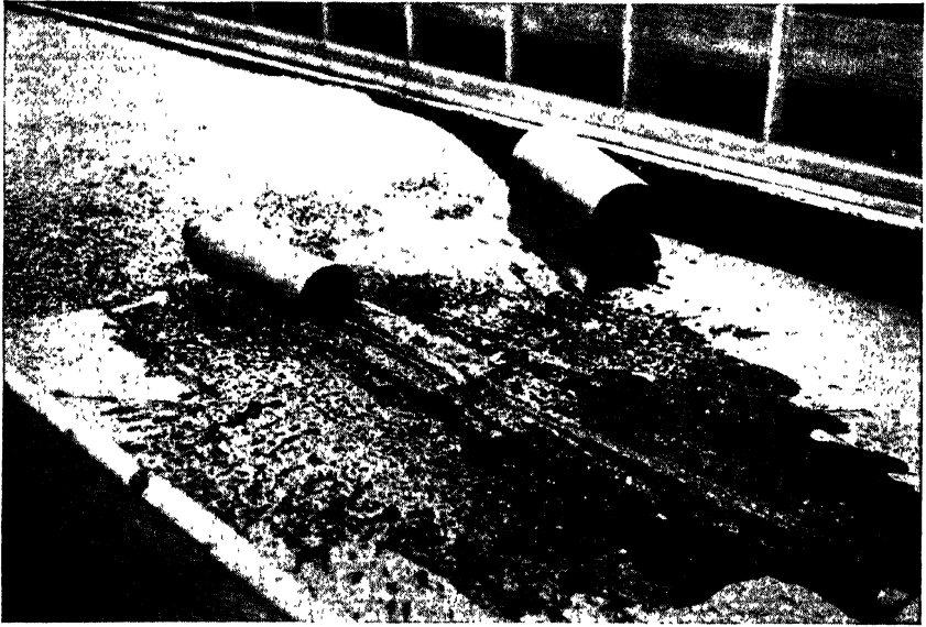
Figure 5-16. Showing placement of half-round tile in bottom of gravel bench, (Ohio Agricultural Experiment Station)
