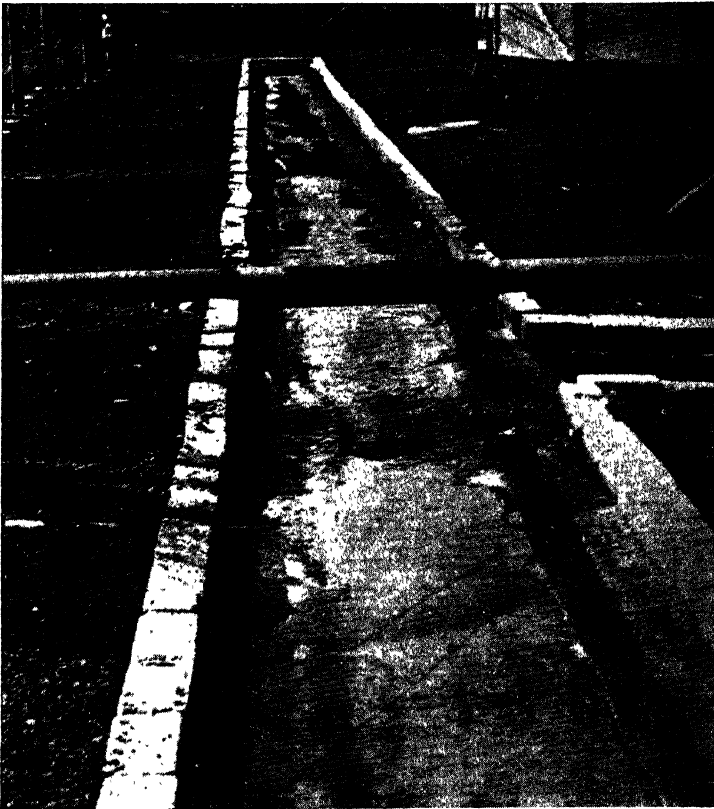
Figure 2-21. Use of asphalt-lined beds and solution drainage trench (shown above) in hydroponics at Ascension Island. (Courtesy U. S. Army, A.A.F.)
