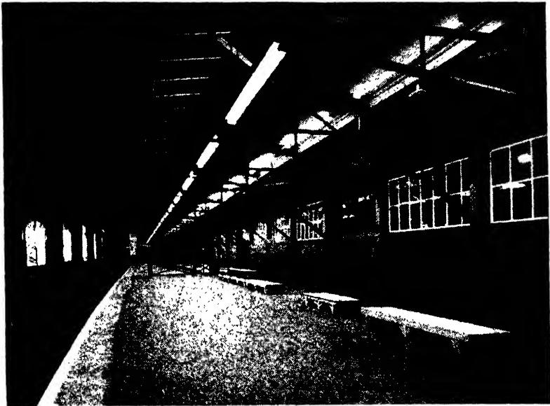
FIG. 42.—Cold Cathode Fluorescent Lighting in Victoria Station. (General Electric Co., Ltd.)
