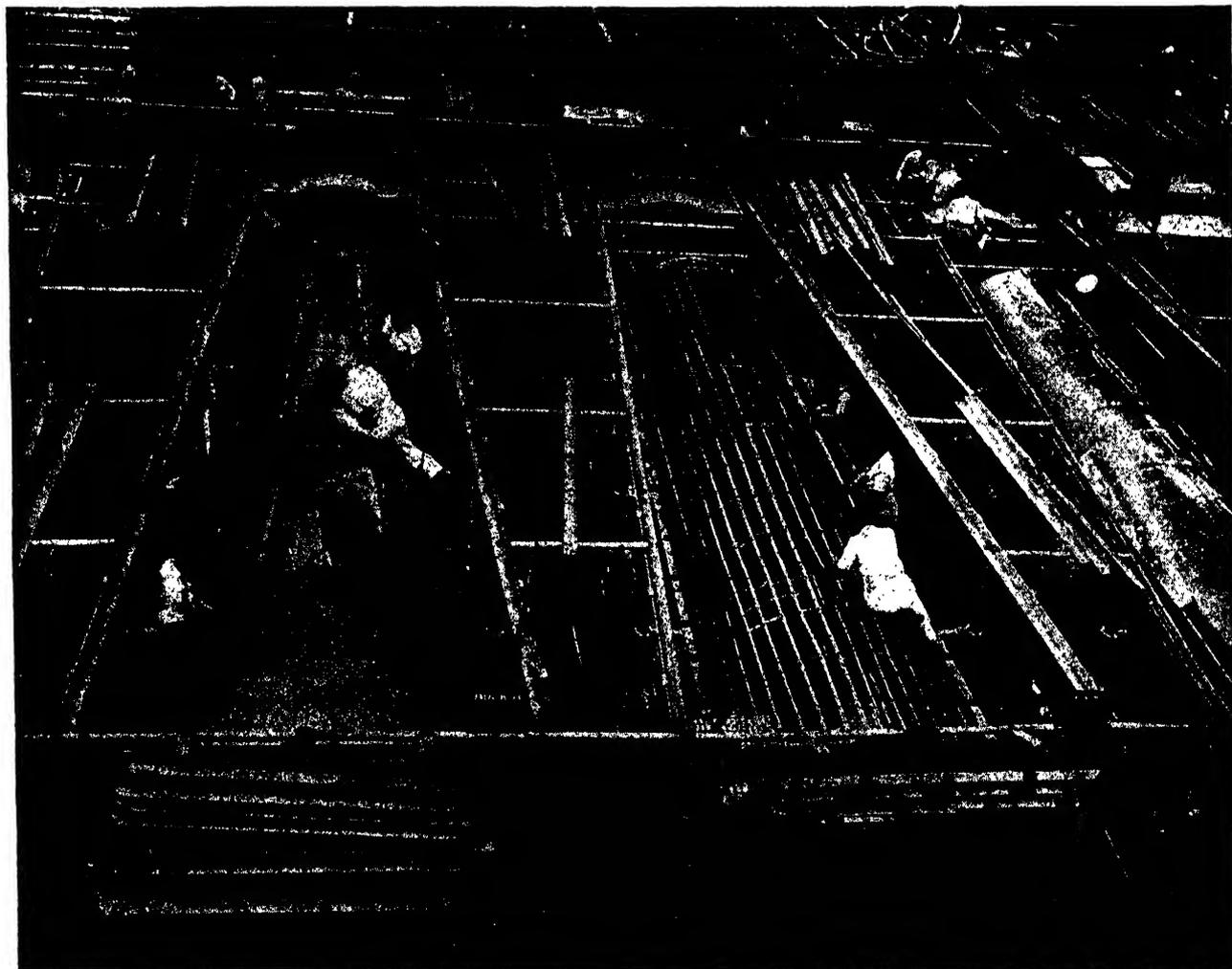
Fig. 287. Aluminum framework and skin being assembled on a Consolidated B-24
