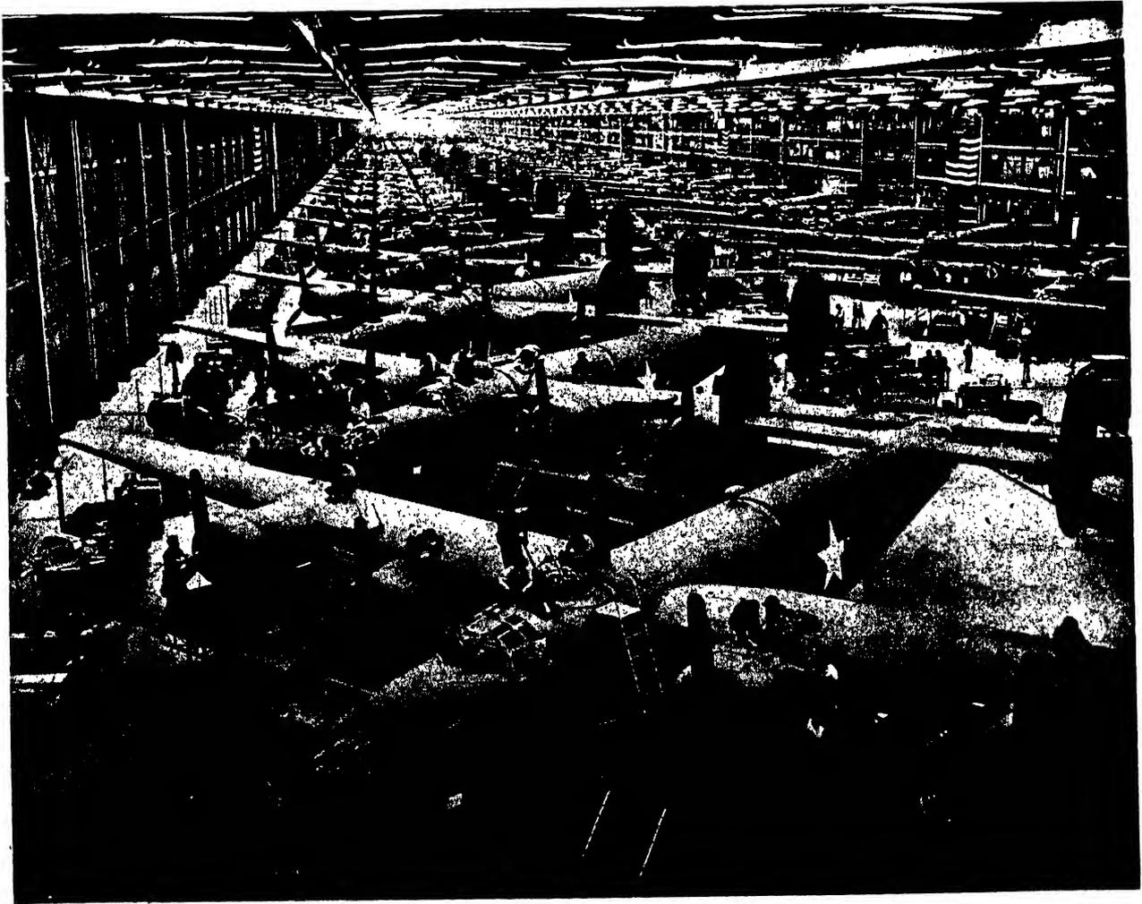
**Fig. 423.** Double assembly line operations during World War II at what was probably the largest aircraft factory in the world, Consolidated's Fort Worth plant. The line in the background contains both C-87 Liberator express transports and B-24 Liberator bombers. The line in the foreground inaugurates assembly line methods of modification to the B-24 bombers.
