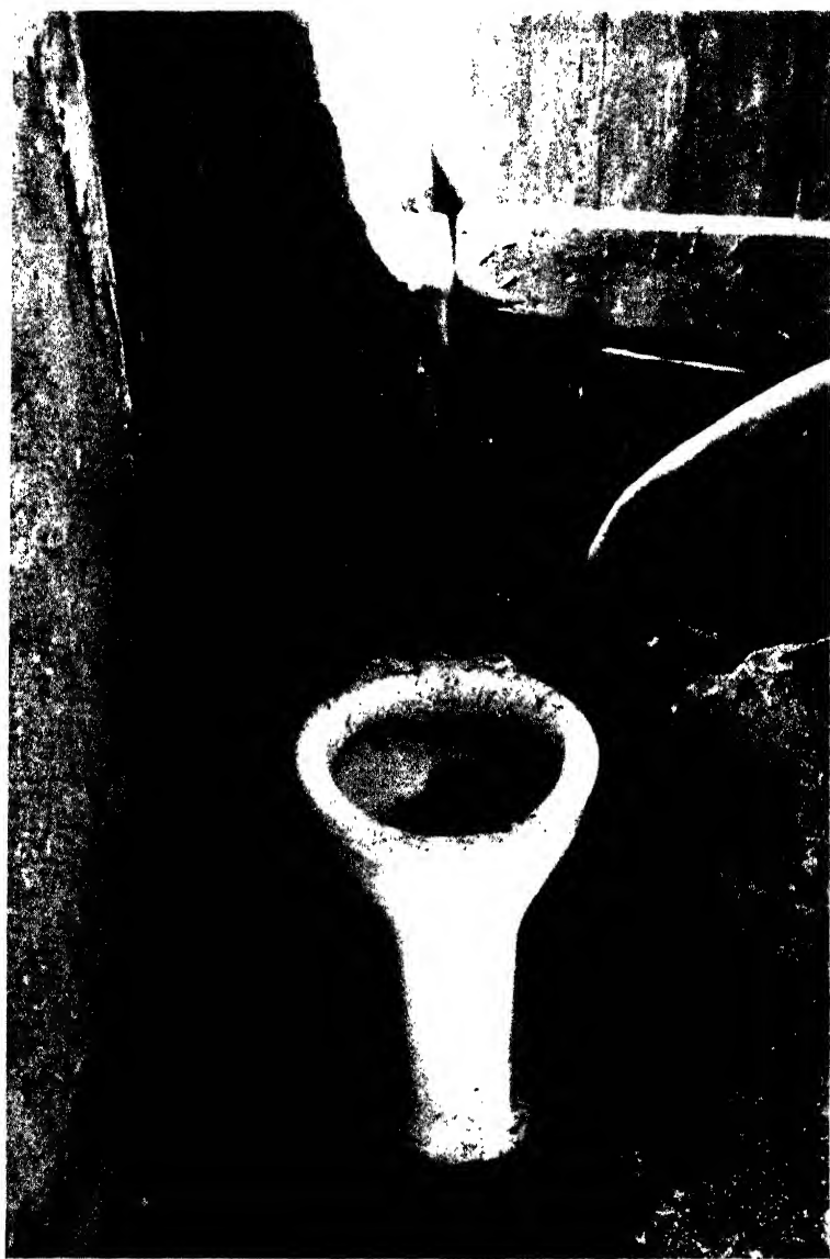
48. The same. Lavatory.
