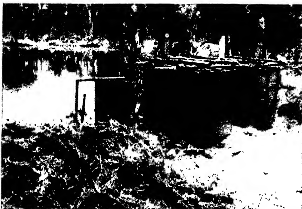
FIG. 32. Production of eucalyptus oil in Australia. A typical distillation post consisting of movable field stills.
