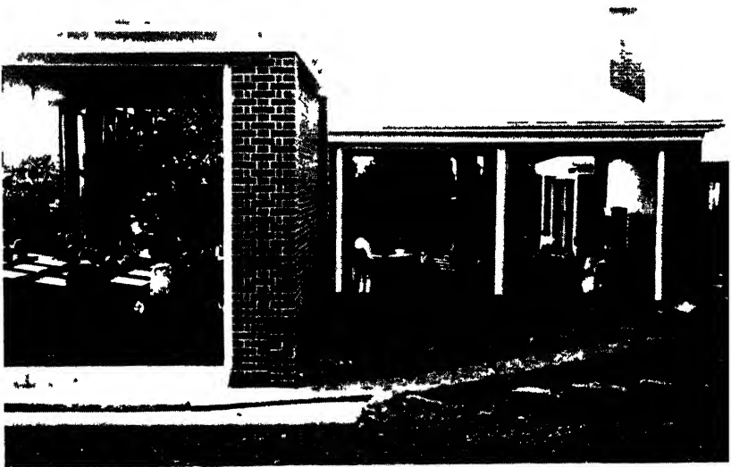
GENERAL VIEW OF THE CLASS ROOMS Uffculme Open Air School, Birmingham.
