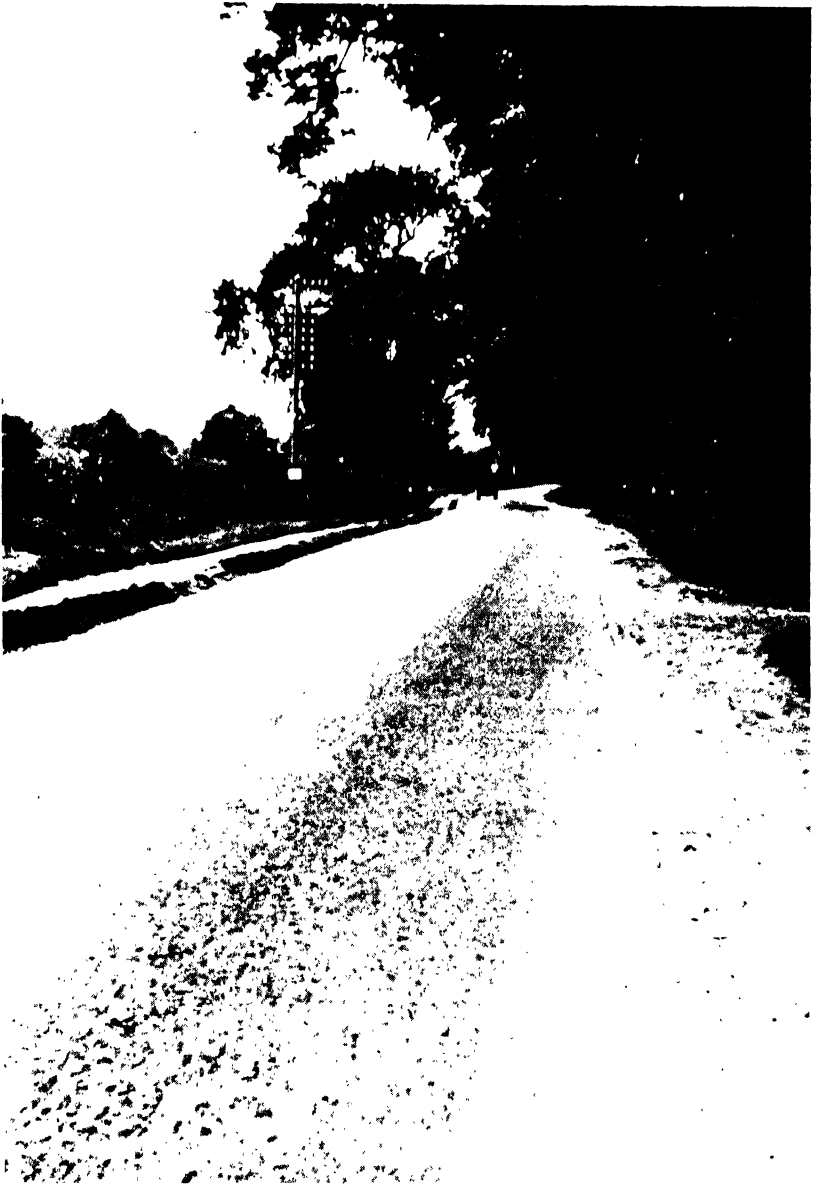
Fig. 21.—Hot Asphalt Limestone Surfacing on A.31 near Altesford. Laid July–August 1930. Photographed June 1945.
