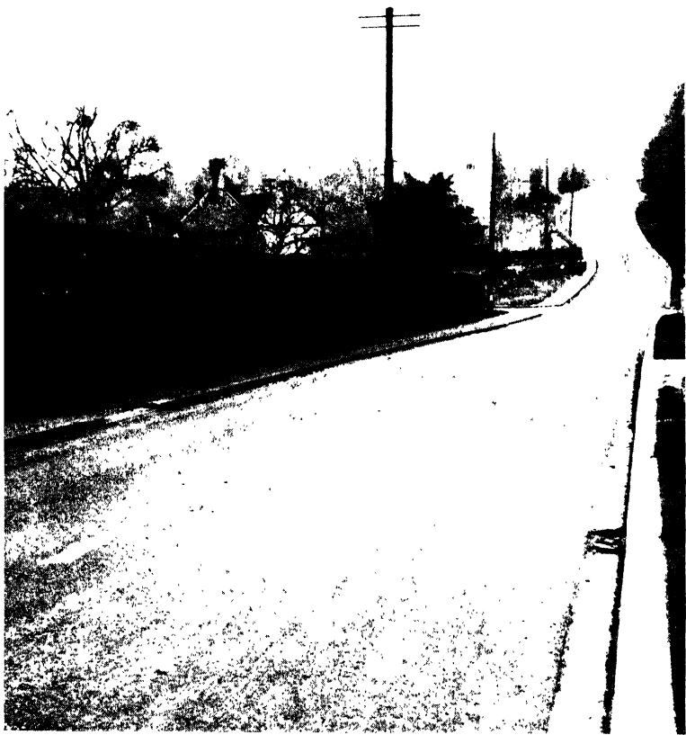
Fig. 20.— \frac{3}{4} -in. Graded Bituminous Carpet (Mountain Limestone Aggregate) laid on A.38 in 1938. Photographed December 1944.
