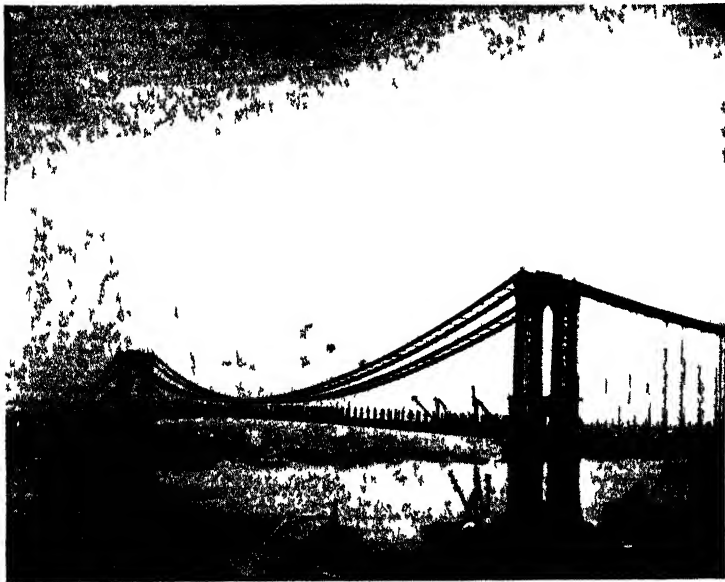
FIG 52—Manhattan Bridge Erection of Diagonals
