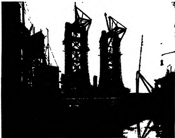
FIG. 45.—Manhattan Bridge. Erection of Towers.
