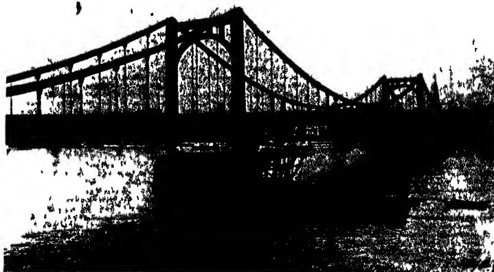
FIG. 17.—Suspension Bridge over the Rhine at Cologne. (Type OS).
