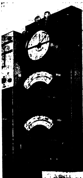
FIG. 1.—SYNCHRONISING BRACKET MOUNTED ON A CONTROL BOARD.
