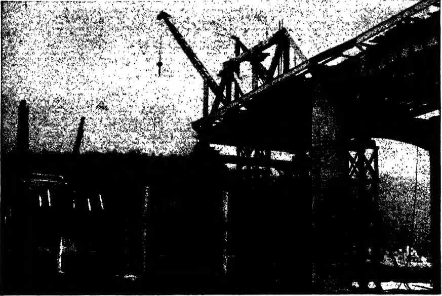
FIG. 13-26A. Construction of the Dravosburg Bridge in Allegheny County, Pa. This is a cantilever bridge. Part of an anchor arm is shown on falsework in the foreground. Notice the simple but neat cylindrical pier shafts. (Courtesy of Parsons, Brinckerhoff, Hall & Macdonald, Consulting Engineers, New York, N.Y. and the Department of Public Works, Allegheny County, Pa.)
