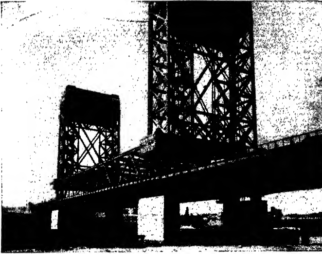
FIG. 13-30. The Stickel Bridge on Route 25A over the Passaic River at Newark, N.J., built by the New Jersey State Highway Department. The piers of the lift bridge were built with pneumatic caissons to rock. One pier base is 60 ft. below mean water; the other, 40 ft. The foundations were designed by Morris Goodkind, bridge engineer, under Spencer Miller, Jr., Commissioner of the New Jersey State Highway Department. The superstructure was designed by Hardesty & Hanover, Consulting Engineers, New York City. (Courtesy of Hardesty & Hanover.)
