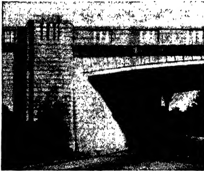
(a) A single-span, concrete, rigid-frame bridge with architectural treatment of surface, and with pylons and U-shaped abutment
