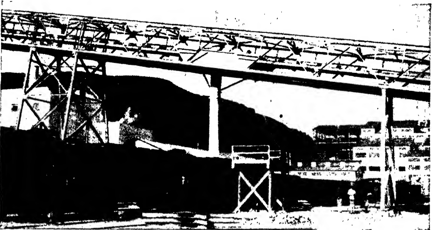
FIG. 8-26. Conveyor trestle under construction at the Morenci Reduction Works, Morenci, Arizona. Notice the single bent and the braced anchor tower. The rectangular chute above the railroad tracks will be used for filling cars. (Courtesy of the Phelps Dodge Corp.)
