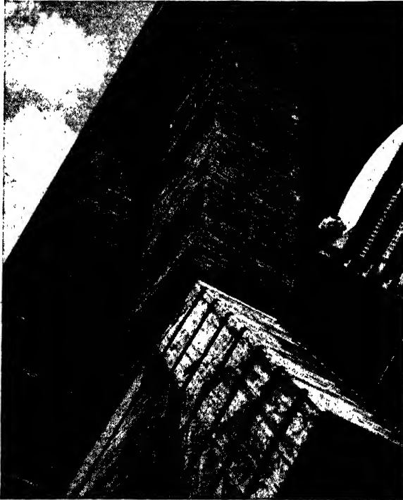
FIG. 14-31. View of a bearing, abutment, and approach piers of the Rainbow Bridge at Niagara Falls, N.Y. as seen when looking upward. Notice the details of the bearing, the fluting, and the rough, ridged surface of the massive piers. (Courtesy of the Niagara Falls Bridge Commission, Niagara Falls, U.S.A.—Canada.)
