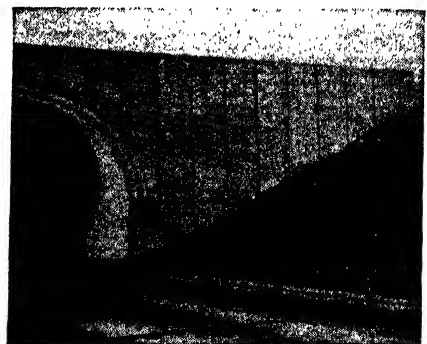
(d) A two-span, concrete, arch bridge with U-shaped abutment and vertical markings
