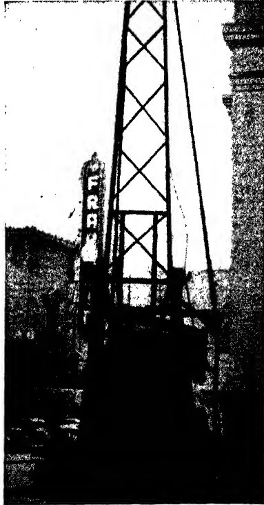
FIG. 3-2. A Raymond Concrete Pile Company's Gow-type wash-boring drill rig. (Courtesy of Dames and Moore, San Francisco and Los Angeles, Calif.)
