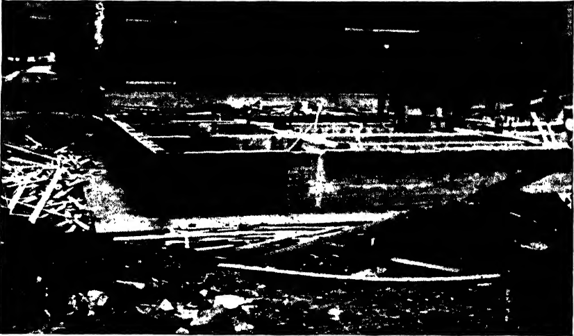
FIG. 7-8A. Ribbed-mat substructures of the Central Mill Boiler House, Anaconda Wire and Cable Company, Hastings-on-Hudson, N. Y. The interior columns will rest upon the ribs at their intersections. The cantilevered portion of the mat will be covered with earth.
