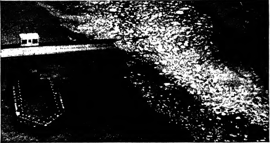
FIG. 13-15A. Air view of bridge over Indian River Inlet near Rehoboth, Del., subjected to pressure of drifting ice. Portion collapsed when a truck and an auto were passing over it, killing three persons and injuring two. (Courtesy of Acme Photos.)
