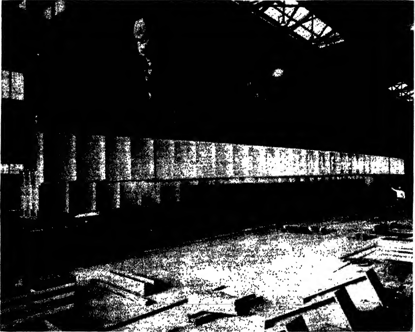
WELDED PLATE GIRDERS FOR NEW YORK STATE THRUWAY (58 IN. DEEP AND 100 FT. LONG).
