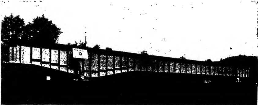
American Bridge Co.
