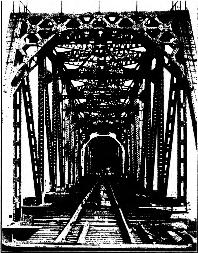
FIG. 46 (j).—Portal of 210-Ft. Span, Louisville and Jeffersonville Bridge, over Ohio River.
