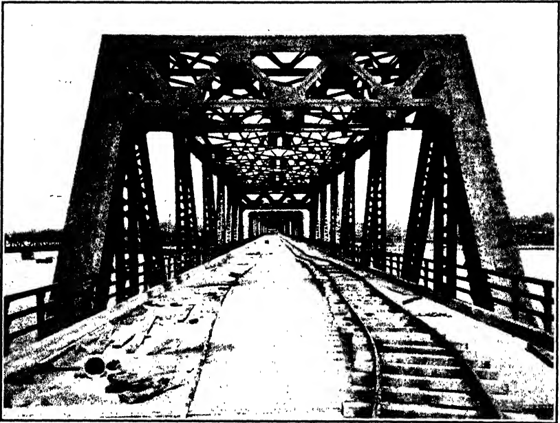
FIG 46 (i).—Portal at End of Main Span at Upper Deck, Mississippi River Bridge, Fort Madison, Iowa.
