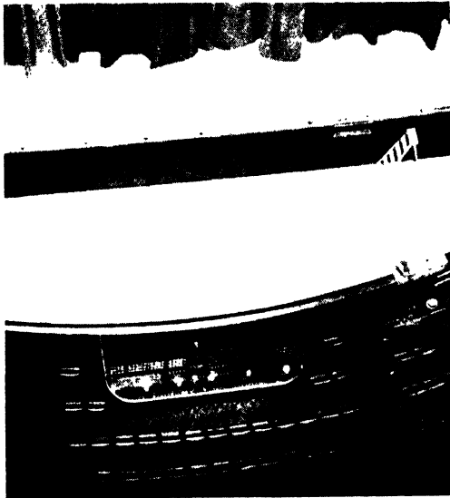
FIG. 100. 314-WAY ELECTRONIC DIMMER CONTROL BOARD: 5-SCENE PRE-SET AND REHEARSAL LEVERS PLUS ACCESSORY CIRCUITS (RADIO CITY MUSIC HALL, NEW YORK, 1933)
