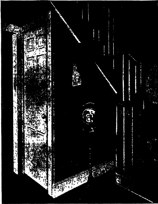
Fig. 91. Open String Stair with Door under the Soffit Courtesy of Curtis Companies, Incorporated, Manufacturers of Curtis Woodwork, Clinton, Iowa
