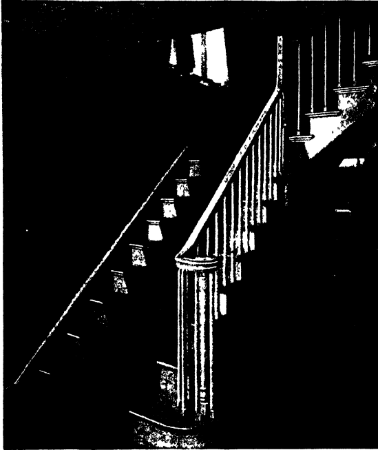
Fig. 8. Stair with Landing about Midway between First and Second Floor (Wide L Stair)
