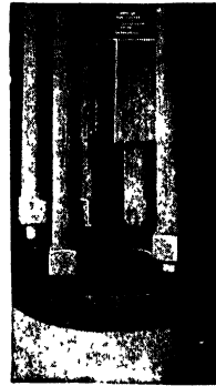
Fig. 99. Lower Ends of a Group of Balusters Showing Dowels which Fit into Holes in the Tread of Bullnose Step
