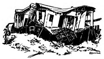
FIG. 85. — House wrecked in San Francisco carthquake of 1906 because the floors and partitions were not securely fastened to the walls (after R. L. Humphrey).
