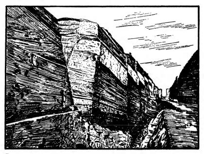
Fig. 41. — Stepfaults in the cutting for the canal across the isthmus of Corinth, Greece. Note offsets of beds.
