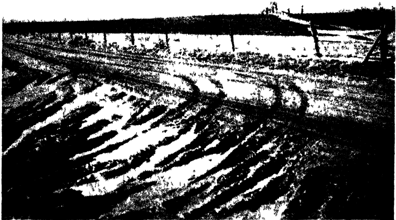
FIG. 182 —View of road in Adams County, Pennsylvania, showing junction of untreated side road with stabilized surface
