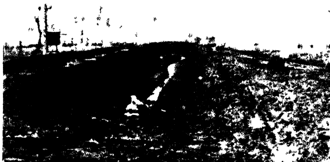
FIG. 128 — Untreated gumbo-soil road in spring of year.
