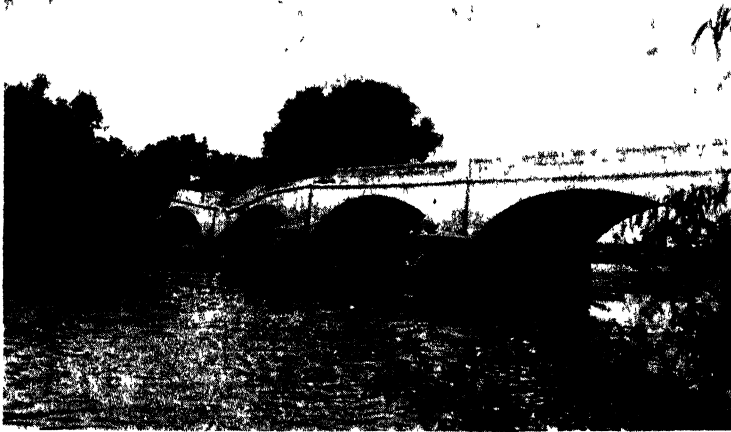
FIG. 75.—Bridge failure caused by settlement of pier.
