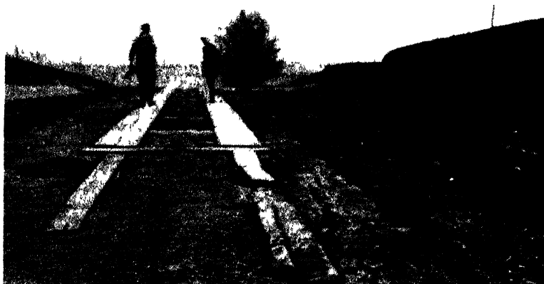
FIG. 66.—Heaved gravel road at beginning of thawing period
