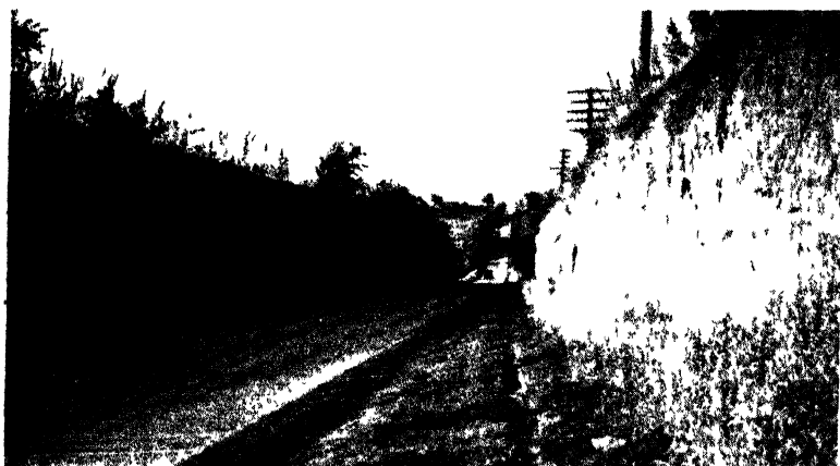
FIG. 72 —Vertical faces of loess soil in cut.
