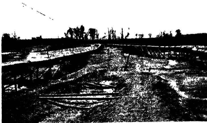
FIG. 168.—Double pipe line for second lift.
