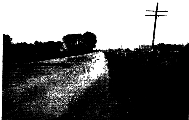
FIG. 69 —Effect of heaving on a gravel road.
