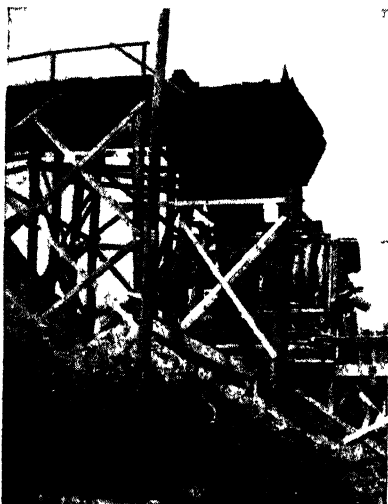
FIG. 139.—Mixing plant for preparation of stabilized-soil road materials.
