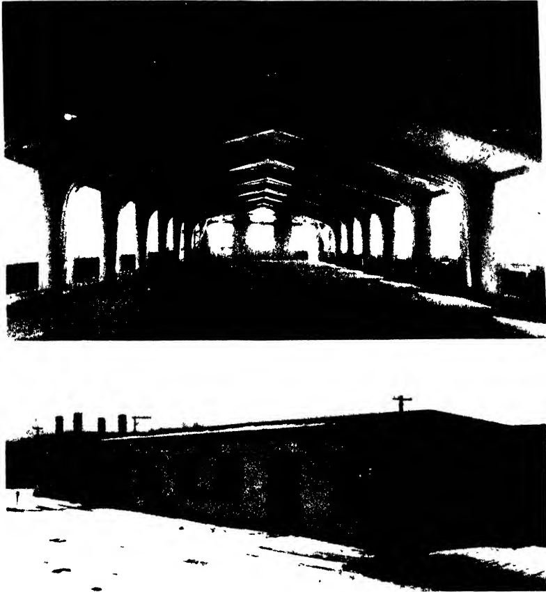
Figure 38.—Use of glued wood construction in garage and storage shed at the Forest Products Laboratory, Madison, Wisconsin. Supporting arches are of laminated wood glued with casein glue. Interior walls are covered with plywood glued with soybean glue. Exterior walls are covered with plywood glued with resin glue and painted after erection.
