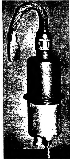
FIG. 4-14. Ignitron. (General Electric Co.)
