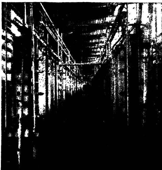
FIG. 122. Hargreaves-Bird cell room. (West Virginia Pulp and Paper Company.)
