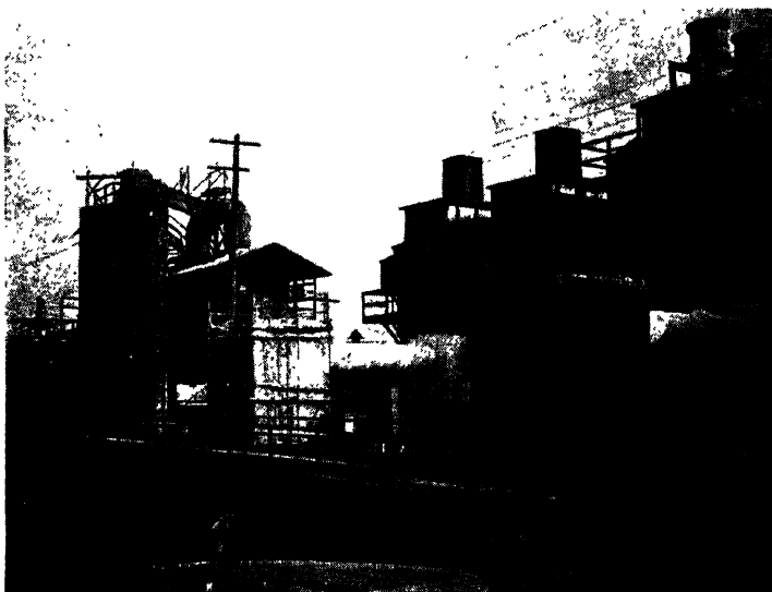
FIG. 239. Hydrators and precipitators for forming H_3PO_4 and preventing its loss. ( Federal Phosphorus Company. )
