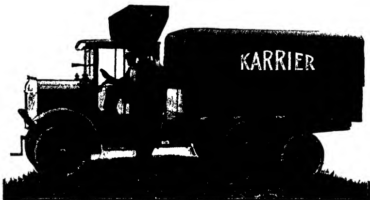
Fig. 16.—Karrier Lorry with Compound Gas Producer
