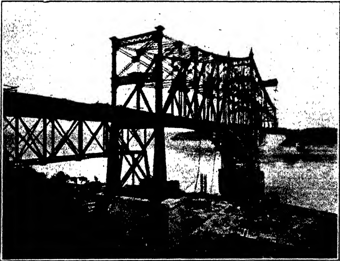
FIG. 61.—Cantilever bridge over the St. Lawrence during erection.
