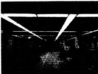
Grid system fluorescent light for machine shop produces broad highlights for reading dials and micrometers.
