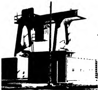
Outdoor installation of vertical pump-motors with switch-gear feature design of this modern pumping station.
