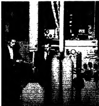
A CO 2 fire extinguisher is checked in the all-weather chamber of the Equipment Laboratory at Wright Field, Ohio, after being subjected to a temperature of -85 deg. F. for 72 hours.
