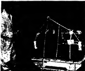
Sharp edges are covered with a soft material and sections of tape, about 20 in. apart, criss-crossed for support. Solution for first application forms spider-web elements that adhere to the tape serving as a base for the wrapping.
