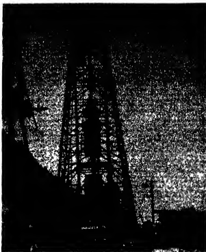
Boring a 6-ft. diameter hole 1,400 ft. deep in Peru, using chilled shot in slot made by cutting tool. Driving apparatus and its operator follow tool down hole.
