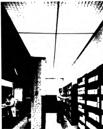
Louverall ceiling using vinylite plastic material in 1" x 2" x 1" openings.
