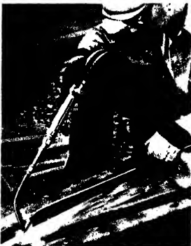
Welding operator builds up frog by the oxy-acetylene process.
