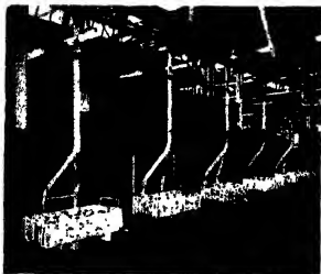
Power centers are best located in the work load area; this saves secondary copper and improves voltage regulation.
