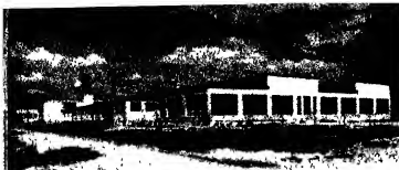
Proper location, adequate lighting and efficient air conditioning characterize this modern mill of the Peppers Mill Co.
