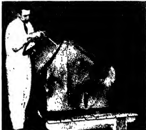
First coating of the plastic cover is applied with an air gun. Yellow in color, it permits the operator to determine uniformity of application. Opening permits gas to escape or provides for ventilation.
