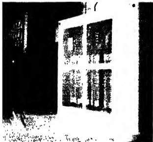
Air cooled dry type transformer, adjacent to switchgear, represents the safest type of unit for indoor operation.
