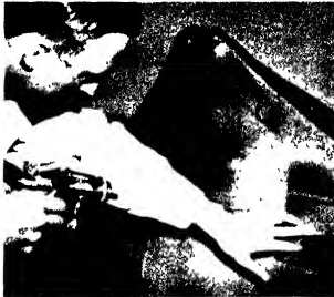
Second coating is red to distinguish from yellow base. The third application generally consists of aluminum paint. When stored under severe conditions, Gilsonite is apphed before painting with aluminum.
