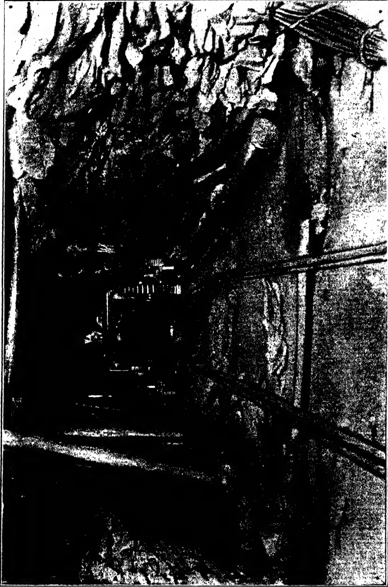
Messrs Clarke & Steavenson's Coal-Cutter at Lidgett Colliery, near Barnsley, in process of "Flitting." This was the first disc coal-cutter adapted to be driven by electrical power.
