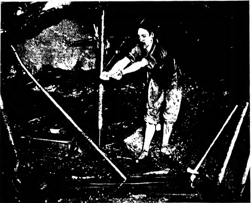
A Stoneman at Work with a Hand-drilling Machine in the face of a Stone Drift.
