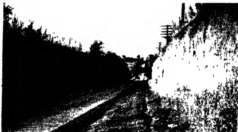
FIG. 72 —Vertical faces of loess soil in cut.
