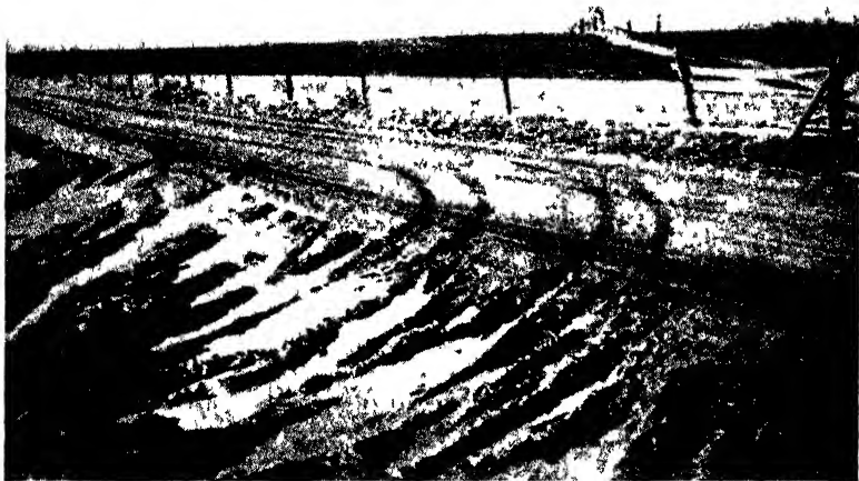
FIG. 182 —View of road in Adams County, Pennsylvania, showing junction of untreated side road with stabilized surface
