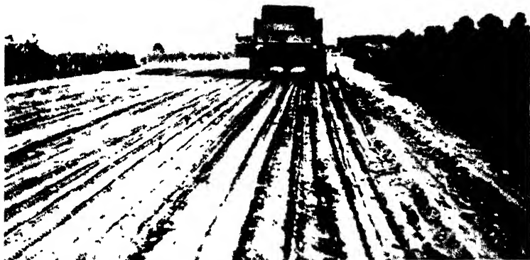
FIG. 148.—Compacting wetted mixture of soil and Portland cement.
