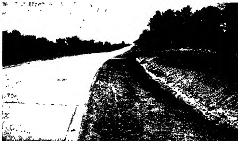
FIG. 161.—Pavement with curb and trough to remove surface water when soils are subject to erosion.
