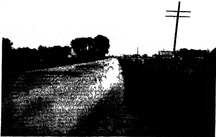
FIG. 69 —Effect of heaving on a gravel road.
