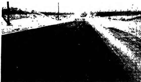
FIG. 151.—Bituminous emulsion stabilized-soil road with surface treatment.
