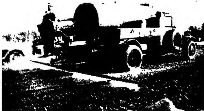
FIG. 147.—Sprinkling mixture of soil and Portland cement.
