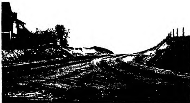
FIG 145 —Intersection of untreated soil road with stabilized road treated with sodium chloride
