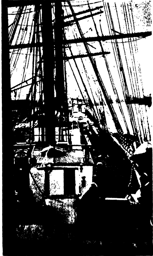
The main deck from the roof of the chart house
