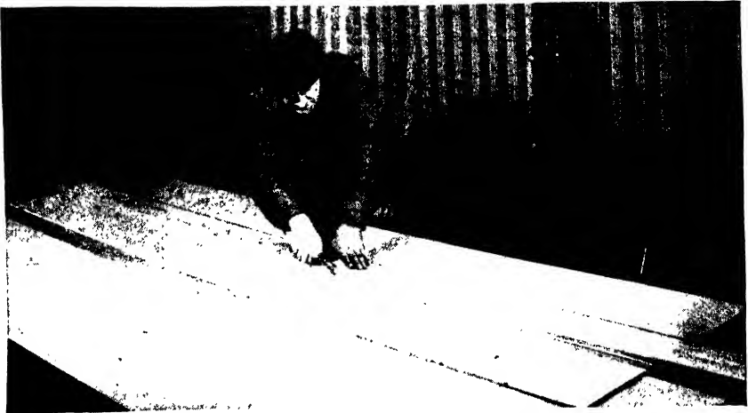
Fig. 11. Workman Scoring Sheetrock Board for Cutting or Breaking Courtesy of United States Gypsum Company, Chicago, Ill.
