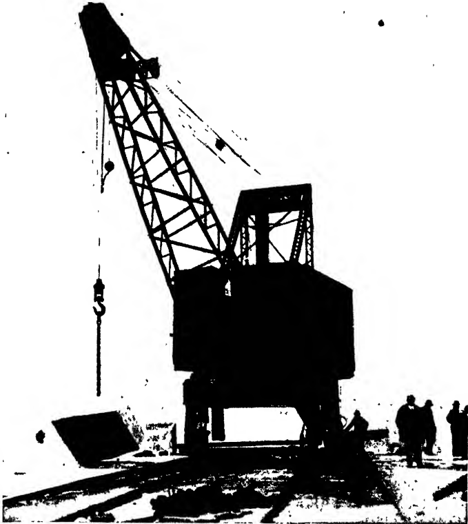
Crane. Illustrates commercial use of the block and tackle. ( Construction Methods. )
