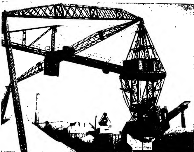
Traveling crane at Merrimac Chemical Company, Everett, Massachusetts, illustrates angular forces. ( Oilways. )
