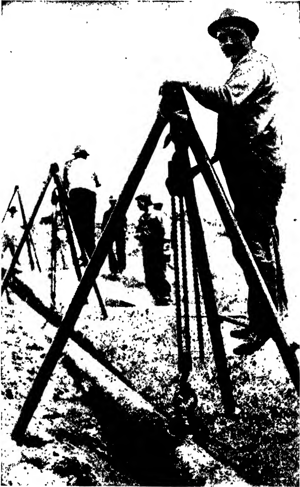
Ratchet lever-type hoist used for handling pipe lines in oil fields. Note the ease with which the workman lifts the heavy pipe. ( Construction Methods. )
