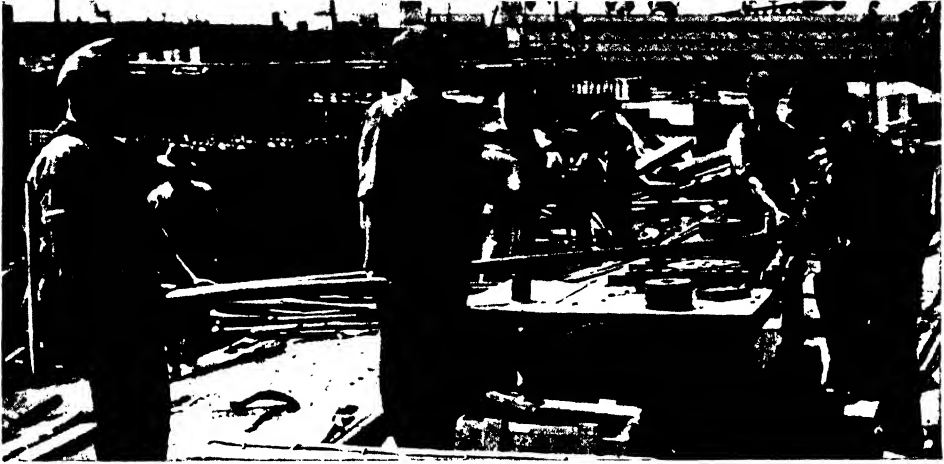
FIG. 64.—BENDING LARGE BARS.
