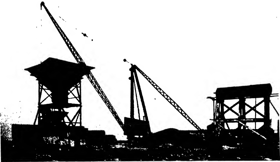
FIG. 37.—AGGREGATE BIN USED IN CONJUNCTION WITH CRANE.
