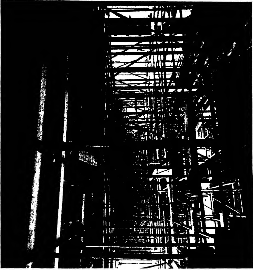
FIG. 263.—STEEL SCAFFOLDING SUPPORTING FLOOR SHUTTERING.
