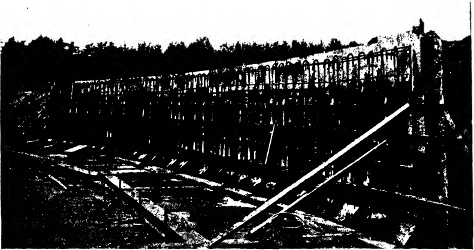
FIG. 364.—STEEL SHUTTERING FOR CIRCULAR RESERVOIR.
