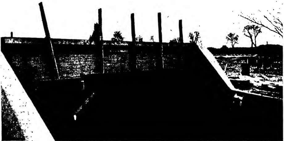
FIG. 313.—SUPPORTING DECK CENTERING WITHOUT MAINTAINING WATERWAY.
