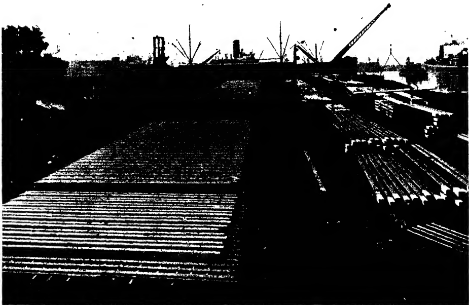
FIG. 9.—TRAVELLING CRANE IN PILE-YARD.
