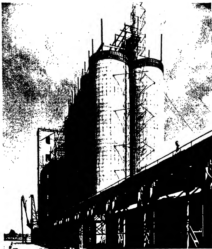
FIG. 151.—HOIST WITHIN STEEL SCAFFOLDING.
