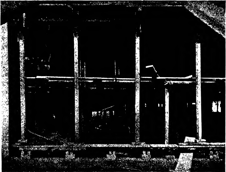
FIG. 259.—TIMBER PROPS FOR FLOOR SHUTTERING.
