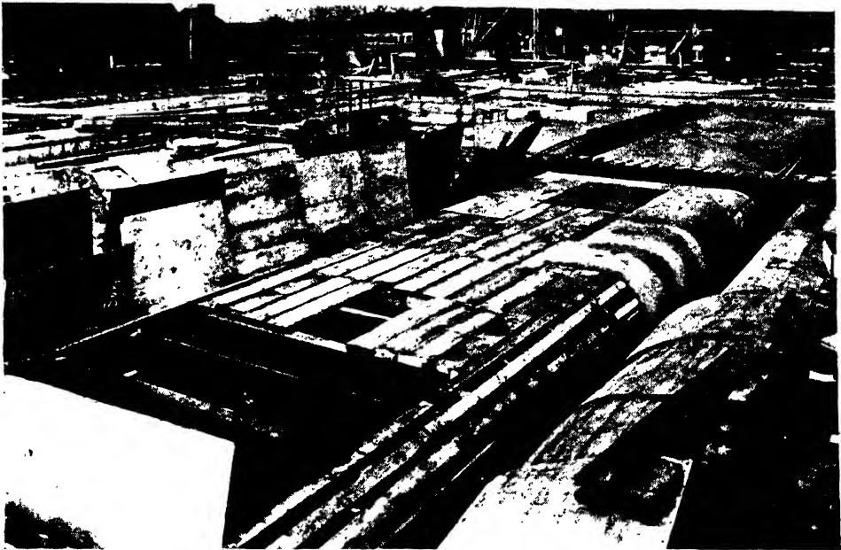
FIG. 104.—PLYWOOD LINING TO CURVED SHUTTERING.
