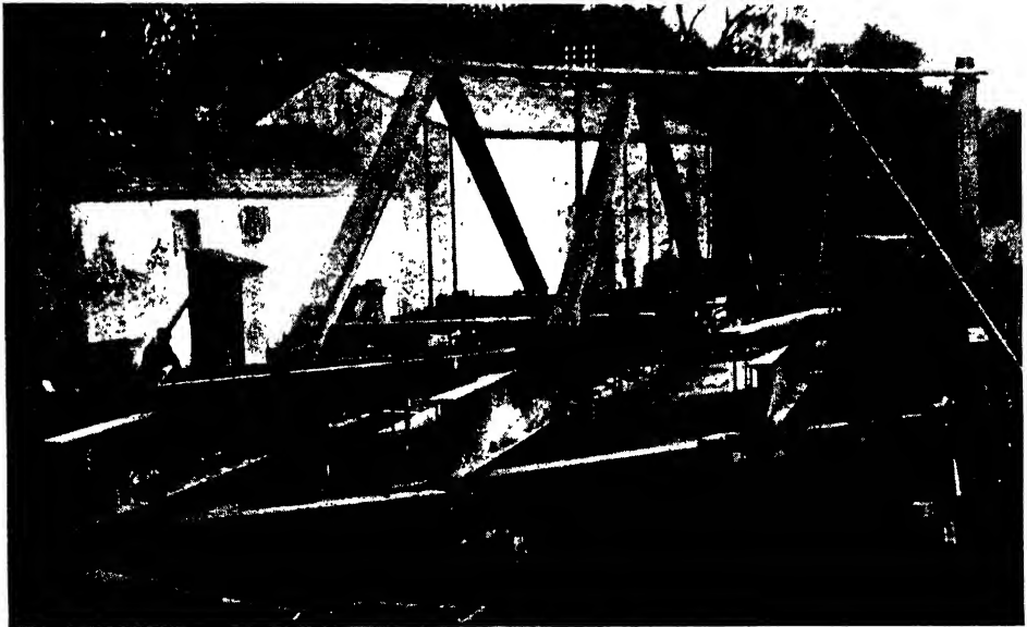
FIG. 315.—SUPPORTING DECK CENTERING WHILE MAINTAINING WATERWAY.
