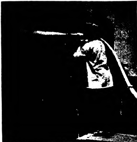
FIG. 394.—APPLYING GUNITE.
