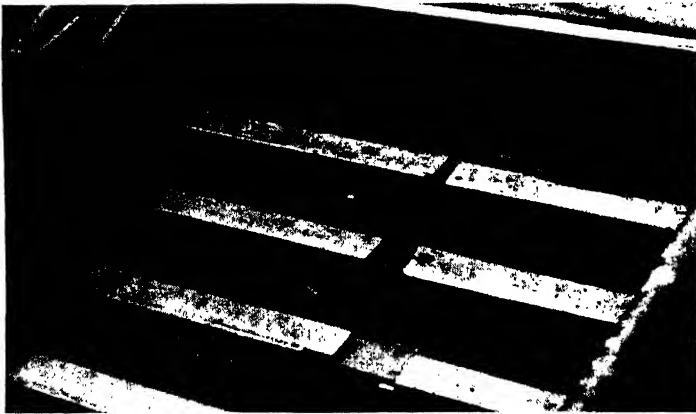
FIG. 176.—PROTECTING STAIR TREADS.
