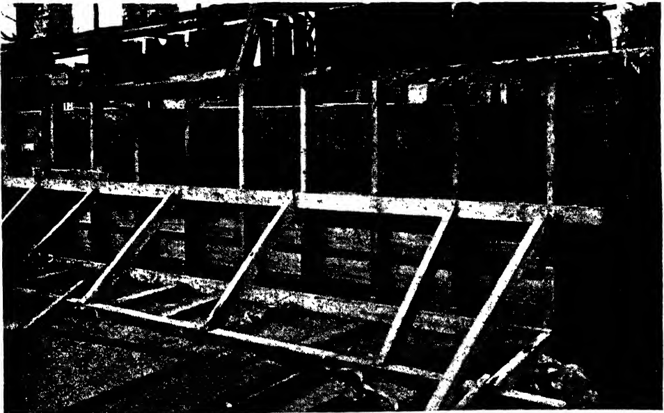
FIG. 105.—SHUTTER LINING.
