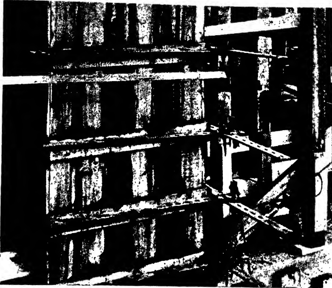
FIG. 113.—STEEL CLAMPS FOR COLUMN BOXES.
