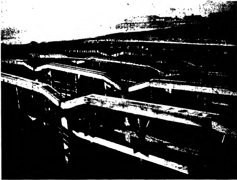
FIG. 277.—HAUNCHED BEAMS.
