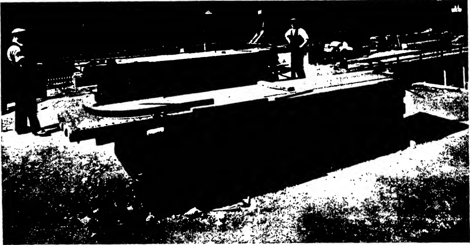
FIG. 61.—BAR-BENDING BENCHES.
