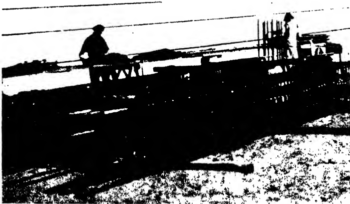
FIG. 81.—REINFORCEMENT SKELETON FOR RECTANGULAR COLUMN.
