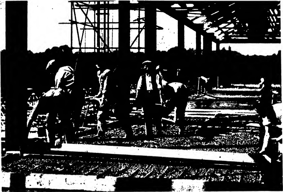
FIG. 279.—SCREEDING SLABS.
