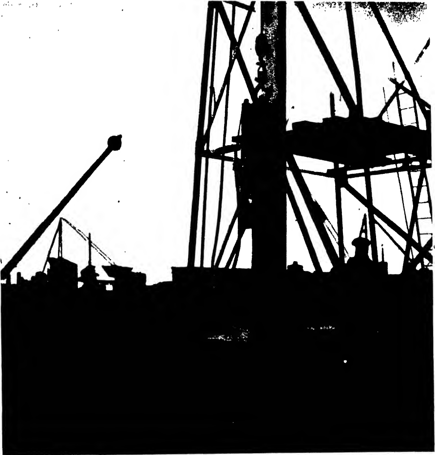
FIG. 200.—DRIVING SHEET PILING WITH HEAVY HAMMER.
