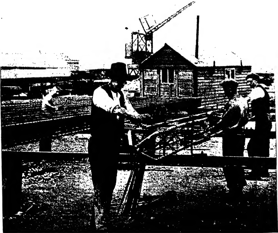
FIG. 80.—ASSEMBLING PILE REINFORCEMENT.
