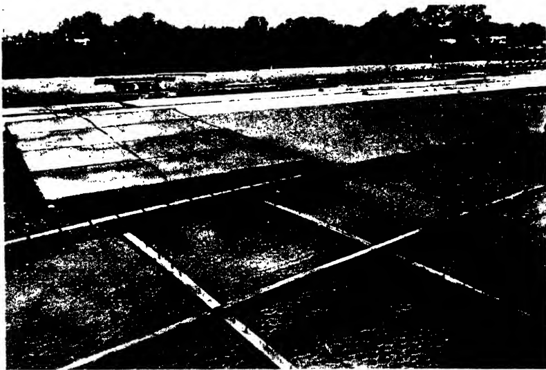
FIG. 174.—COCO-NUT MATTING ATTACHED TO FRAME.
