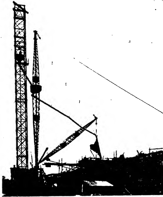
FIG. 155.—CHUTING PLANT.
