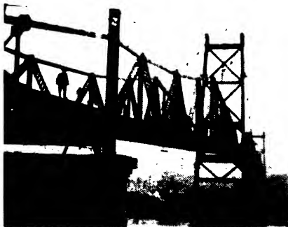
I-bar suspension bridge
