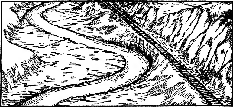
FIG. 92.—A railroad in Central America undercut by a stream.
