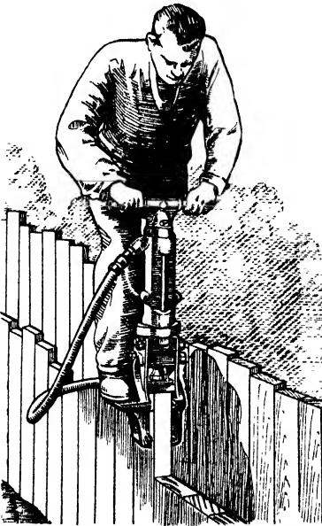
Fig. 8. —SHEETING DRIVER DRIVEN BY COMPRESSED AIR
