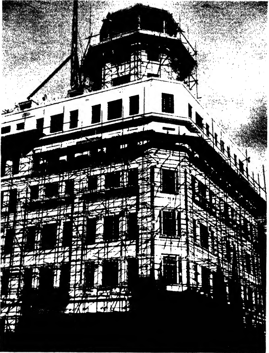
Fig. 1. —STEEL SCAFFOLDING IS AN INDISPENSABLE ADJUNCT TO MODERN BUILDING OPERATIONS
