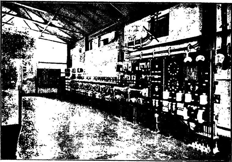
Fig. No. 9. Karjat Traction Sub-Station—Control Room.
