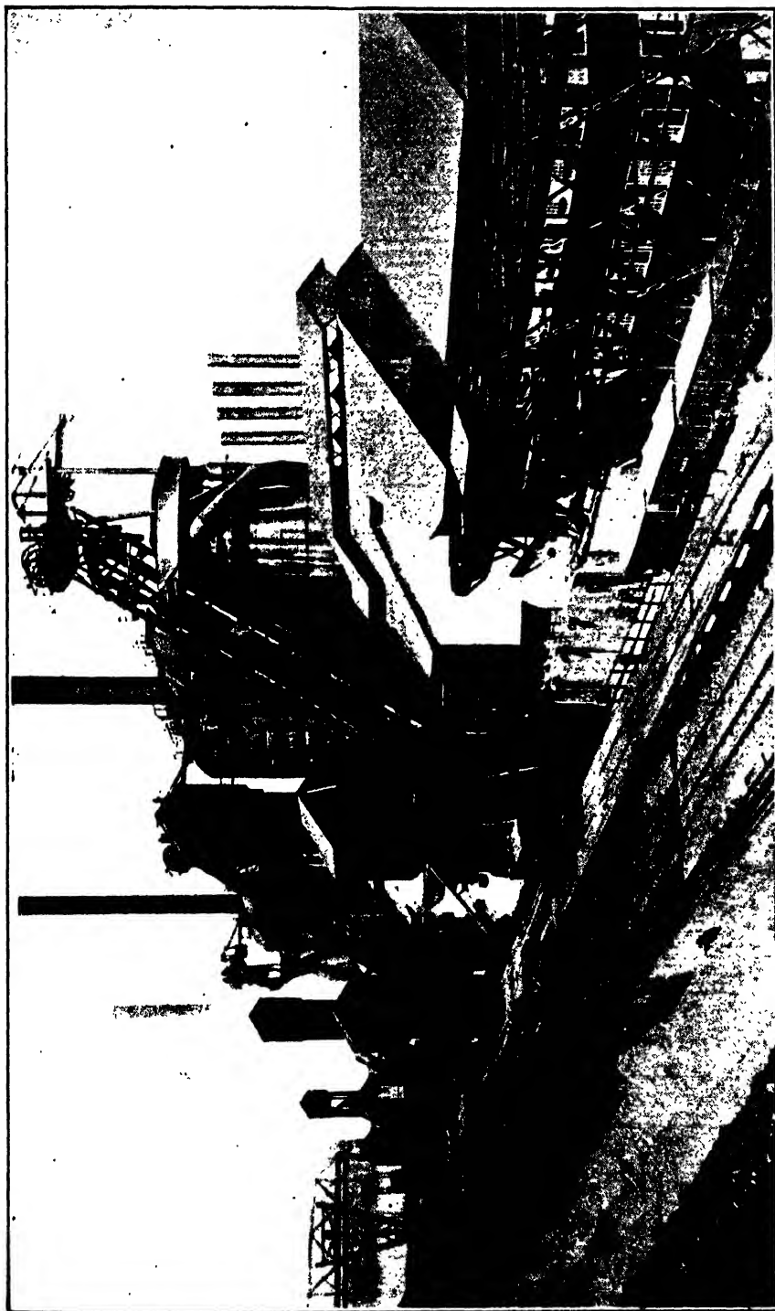
FIG. 109.—A modern iron-smelting plant. The stock pile of ore may be seen at the left, and above it the traveling crane used in loading the small cars which move up the inclines to charge the furnaces. (Courtesy of the Iron Trade Review, Cleveland, Ohio.)
