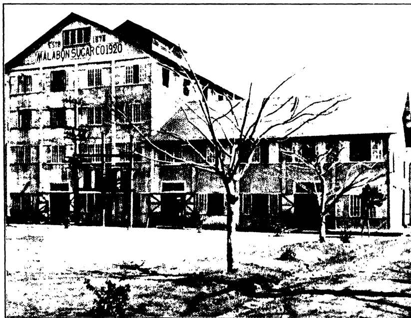
BUILDINGS OF TROPICAL NORIT REFINERY IN THE PHILIPPINES.
