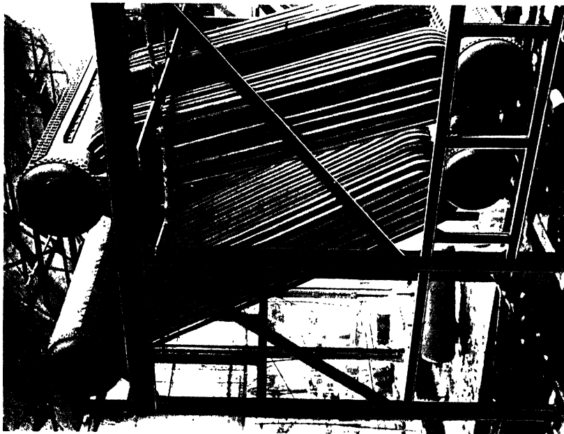
BOILER IN COURSE OF ERECTION IN BRITISH INDIA. (John Thompson Water Tube Boilers, Ltd.)
