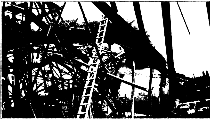
BAROMETRIC CONDENSER TUMBLED OVER DURING A CYCLONE.
